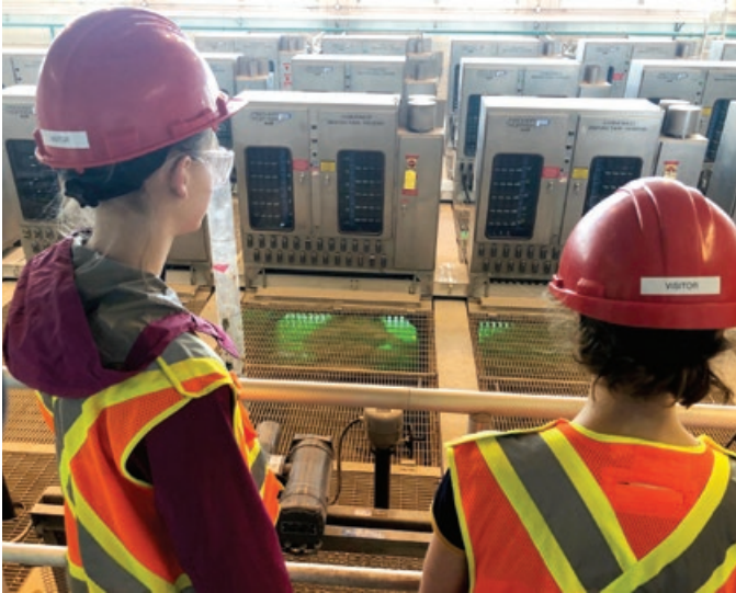
TOURING A WASTEWATER TREATMENT PLANT IS AN EYE-OPENING EXPERIENCE
